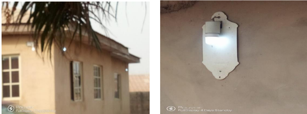
Fig 2: Power wastage through lighting during daylight
