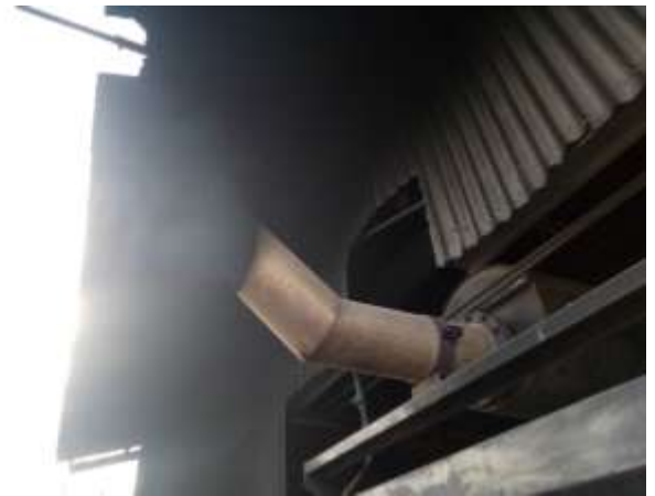
Fig. 30 Exhaust System of the Diesel Engine
