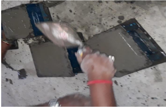
(b) Smoothing the top layer of mix
