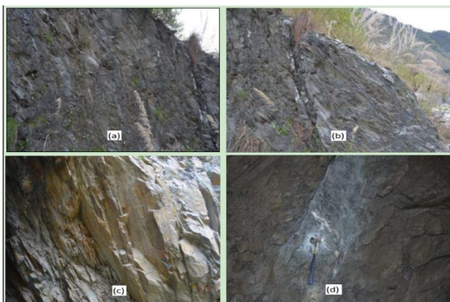
Fig. 2. Showing various Geological characteristics.(a) kink bands in SP occupied zone (b) Distressing in SP band at surface. (c). Swelling and pinching shear zone filled with clay gauge. (d). Shear zone in PQT+PQM occupied area.
