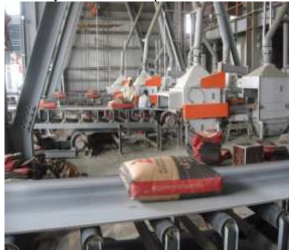
Figure 1 Atbara Cement Factory
