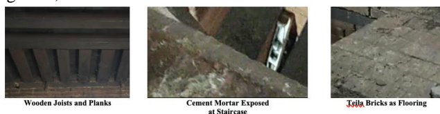
Fig. 4. Section of Flooring
