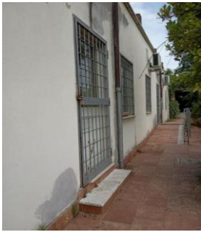
Fig. 6 Building's exterior situation
