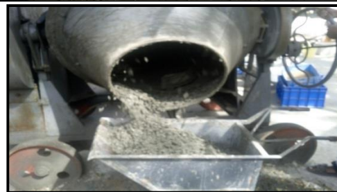
Fig.2 .Mixing Of Concrete
