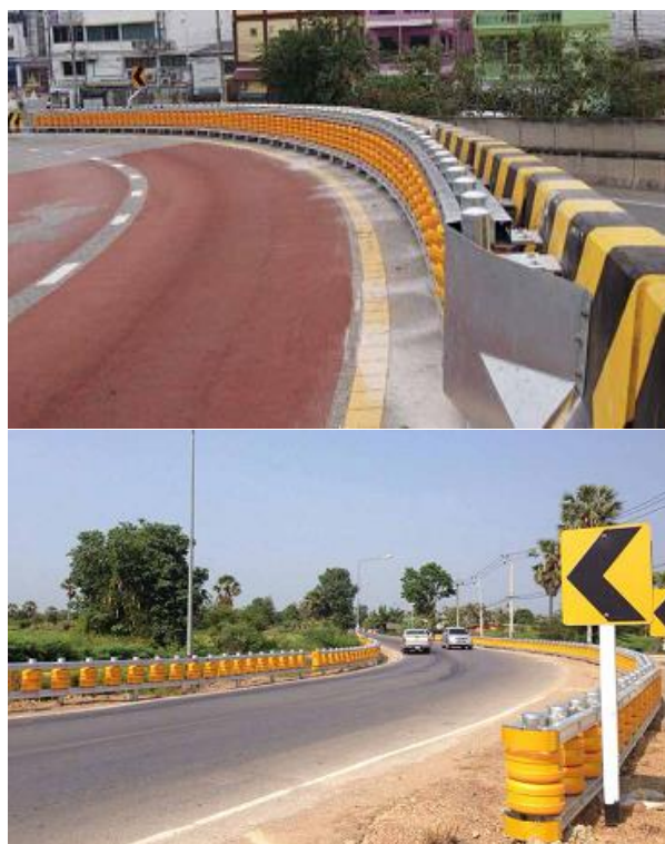
Fig. Installation of barriers on existing barriers & new barrier construction
