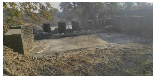
Fig.5. Foundation construction phase showing reinforcement layout
