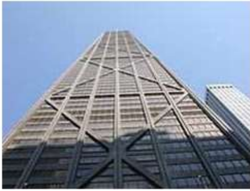
Fig 2.3 Cross - diagonals
