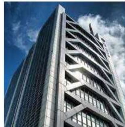
Fig2.6 Eccentric bracing
