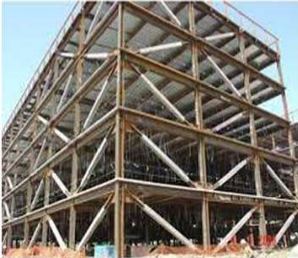
Fig 2.7 Buckling Restrained Brace
