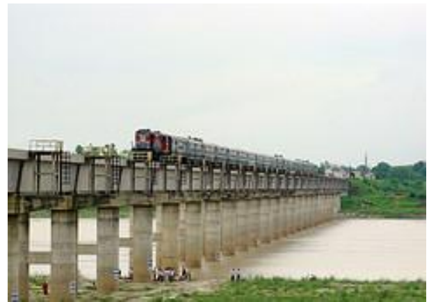
Fig. 7 Train is on River Bridge
