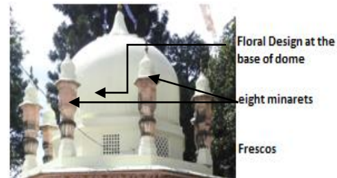
Fig.20 Dome at Samadhi
