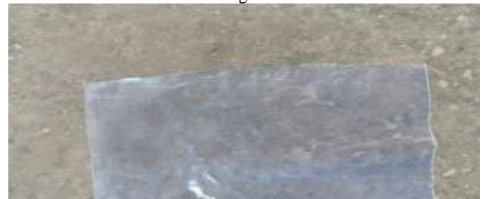
Figure .03 Liner mouth defect
