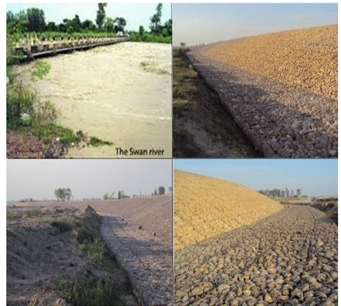
Fig. 4. Completed embankment in Phase-II
