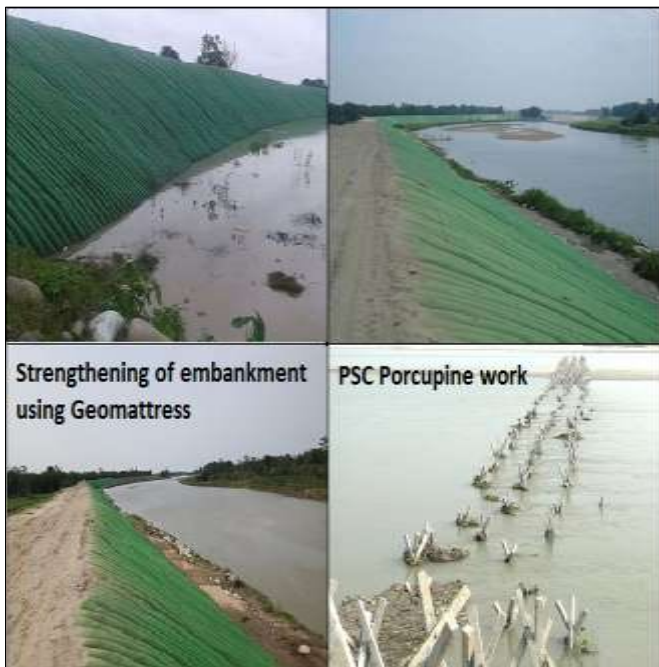
Fig. 7. Implementation of geotextile mattress and porcupine works
