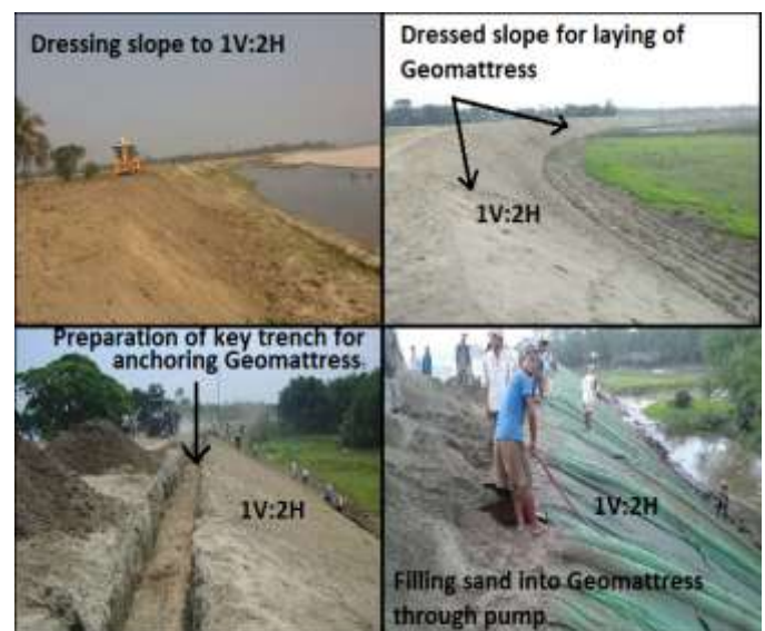
Fig. 5. Installation of Geotextile mattress at various stages
