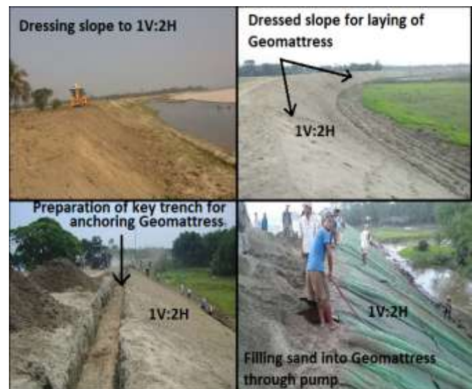
Fig. 5. Installation of Geotextile mattress at various stages
