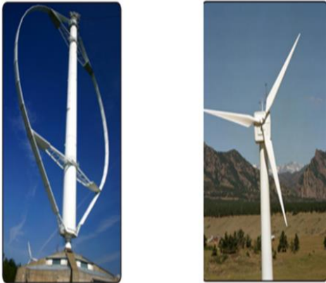
(a) Vertical axis wind turbine (b) Horizontal axis wind turbine
