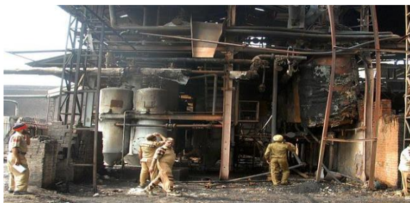
Fig 1: Workers Working In Polluted Environment
