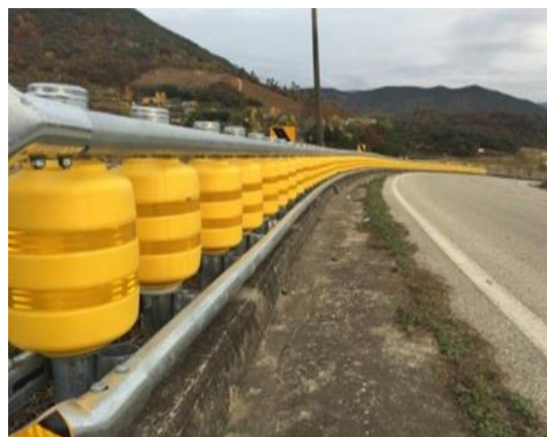
Fig. Rolling Barriers on horizontal curve
