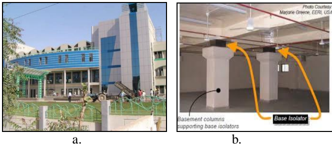
a. Bhuj Hospital Gujarat, India. b. Seismic Rubber Bearing.
