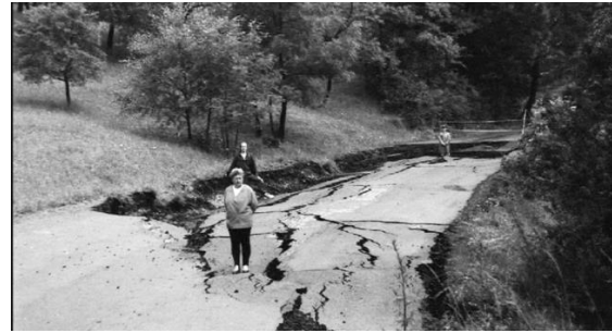
Fig. 8. Example of damage to a road by a landslide in the village of Halenkovice in July 1997 when the road embankment subsided by 1 m. Photo A. Horká.
