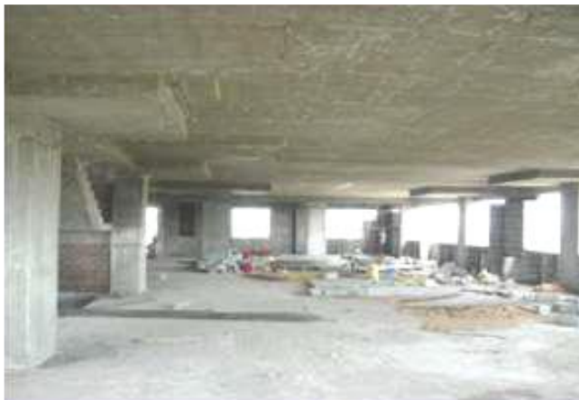
Fig. 3. Flat Slab (with drop).
