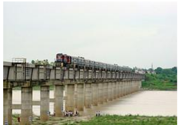
Fig. 7 Train is on River Bridge
