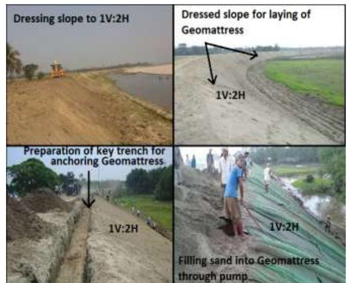
Fig. 5. Installation of Geotextile mattress at various stages
